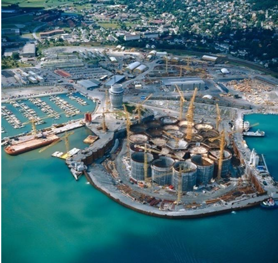
Hinna Dry Dock 1986. GFC 42 m tall in a 14 m deep dock. Float-out on giant air cushion
