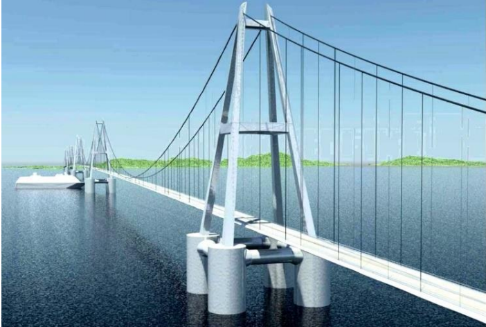
Suspension bridge on floating pontoons
